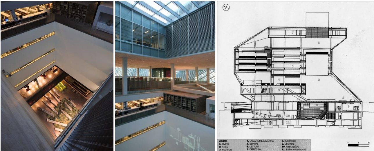
Figure 1. Atrium of the Seattle Central Library which uses vertical space to enhance the stack effect ( https://en.wikiarquitectura.com/building/seattle-public-library , 2024)
