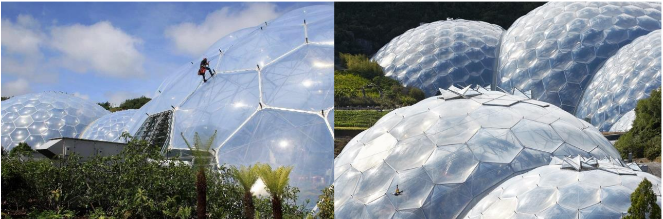
Figure 3. The Eden Project in the UK uses ETFE foil cushions allowing high light transmittance and insulation (Archdaily, 2024).
