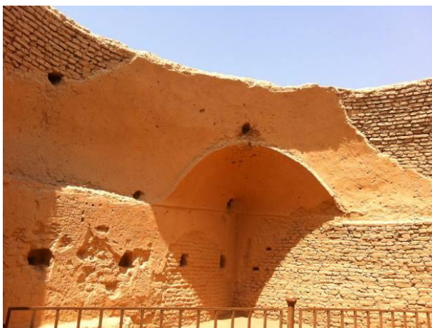
Figure 10. Adobe Brick Construction
