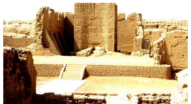
Figure 6. Central Tower Hall
