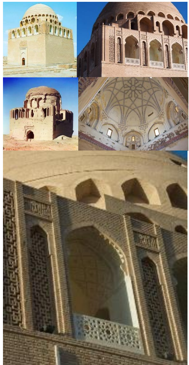
Figure 5. Mausoleum of Sultan Sanjar reflects innovative technology, integrating Hazārḡāf brickwork, tile revetment, and painting into a unified structure with symbolic depth. (Photos: authors' archive).
