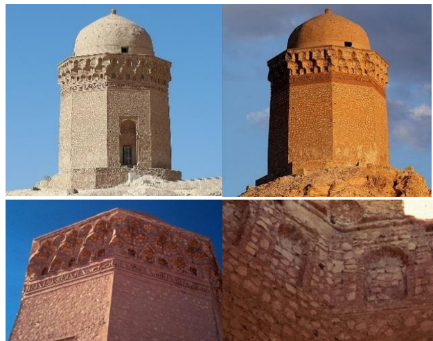
Figure 2. Gunbad-i ‘Ali refines Proto Technology, with its cylindrical tower and conical roof in plain brick, enhanced by texture and Kufic inscriptions, emphasizing material and form (Photos: authors' archive).
